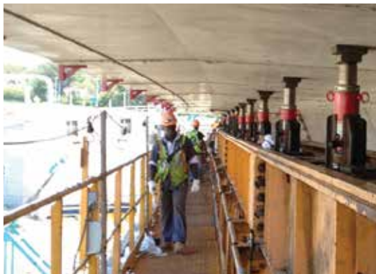
(42) HLN5508 lock nut cylinders lifting the Jordan Bridge in Chesapeake, VA.
